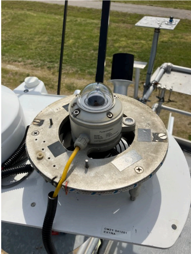
Photo of a pyranometer mounted on a sun tracker. Note connector position.
