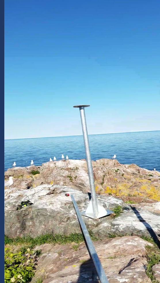
2 large posts installed in granite rock with anchor bolts. Solar tracker and AERONET cimel secured on top of circular mounts
