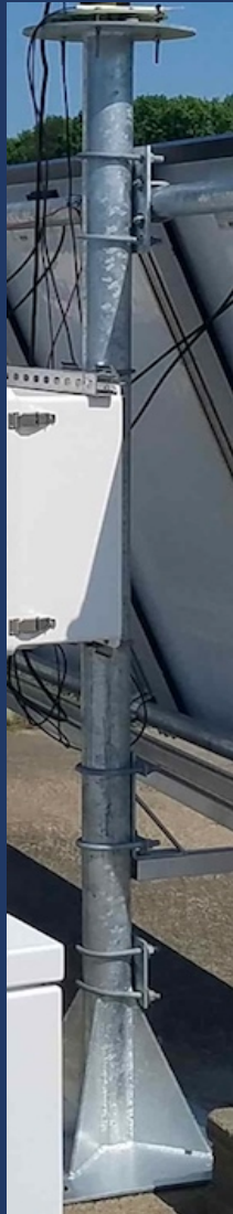
Hot-dipped galvanized post
